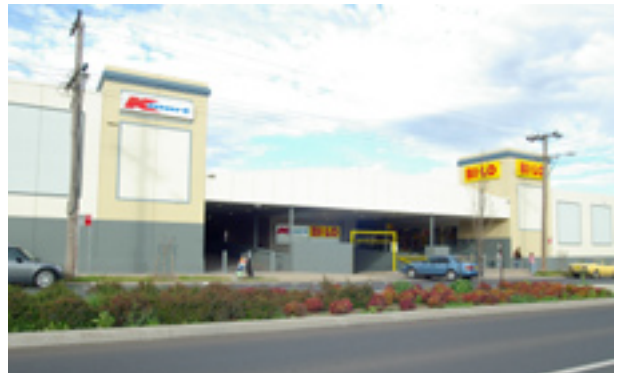
Parkes Shopping Centre Stage 2, Parkes, NSW
