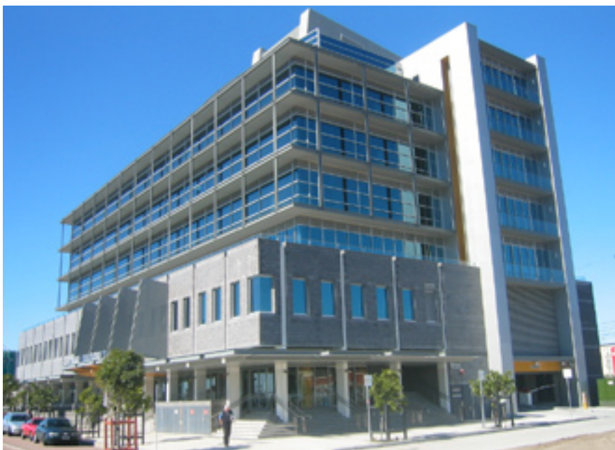
Honeysuckle House Stage 1, Newcastle, NSW
