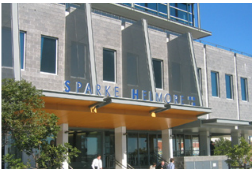
Honeysuckle House, Stage 1 (Newcastle, NSW)
