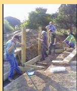
▲ Volunteers building the jump
