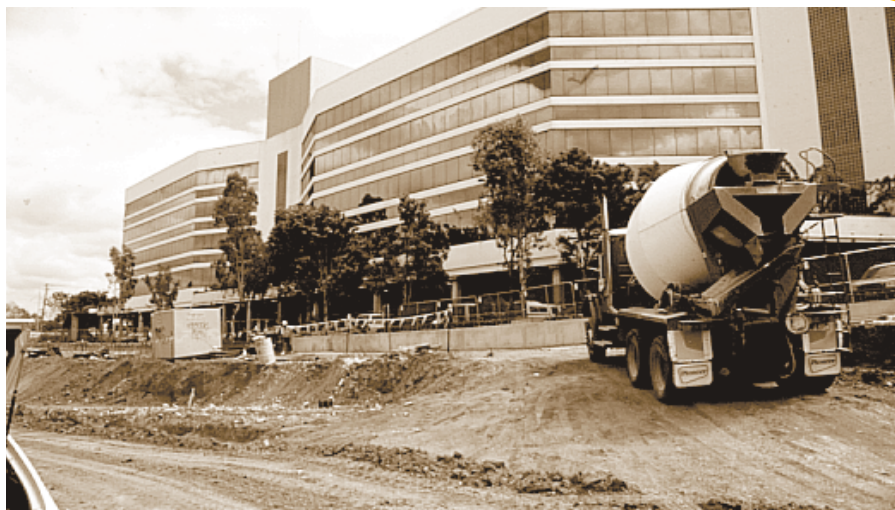
South East Transit Busway works adjacent to Garden Square Office Park
