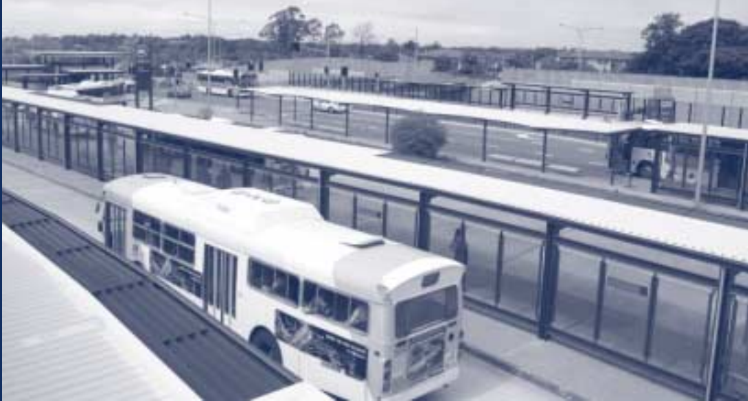
New South East Busway interchange facility at Garden City.
