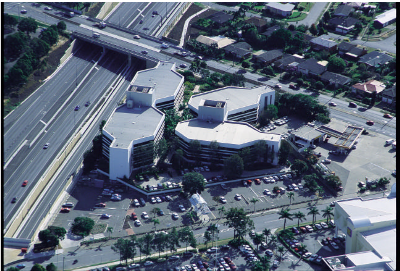
An aerial view of the Garden Square Property
