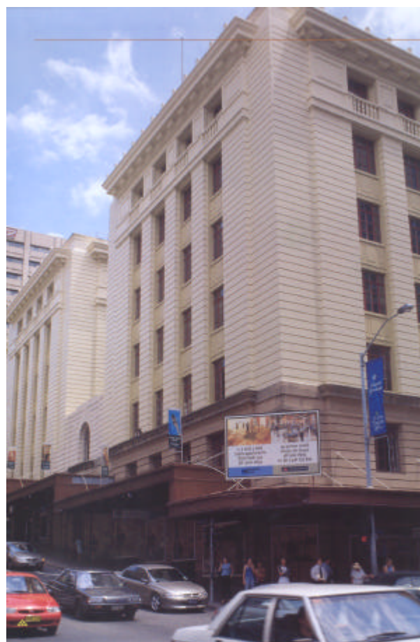
The two low rise towers of the Anzac Square complex in which the Anzac Square Offices are located
