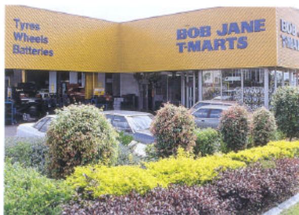
The Bob Jane T-Marts building fronting Kessels Road
