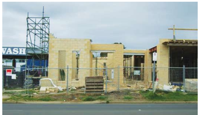
▲ Cowes Branch under construction.
